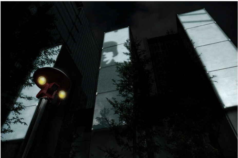
Fig. 6.4. Christian Möller’s interactive facade on the Osaki Building Tokyo 2006
